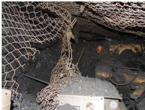
Fig. 2. Deformation of the roadway caused by a rockburst.
